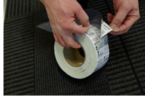
A.1 Peel the TileTab from the roll
